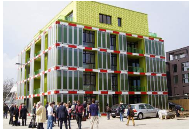
Colt joined with Arup and SSC to create the Bioreactor Façade, a dynamic façade system for the production of renewable energy using algal biomass and solar thermal heat, here shown in its prototype house in Hamburg
